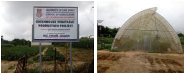
Installed greenhouse at AG Carson Technology Village, UCC
