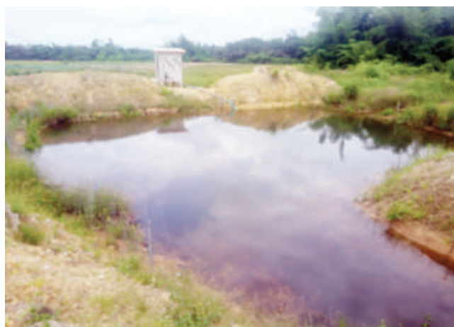
Irrigation pond and pump station
